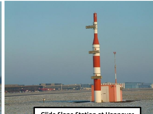
Glide Slope Station at Hannover
